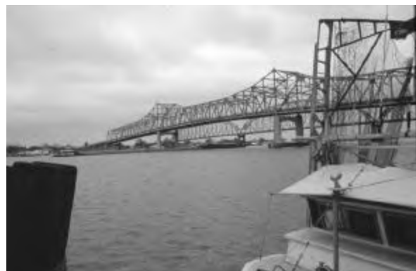
Figure 3.8. The bridge leaving Morgan City
